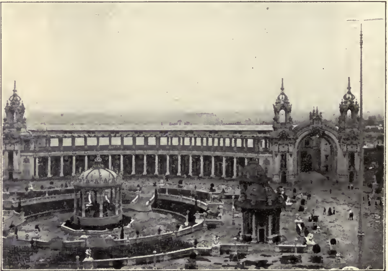
SUNKEN GARDEN BEHIND ELECTRIC TOWER
